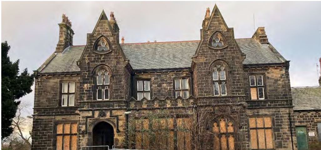
Micklefield House, awaiting conversion
